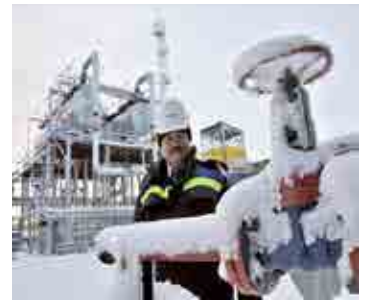
Gas treatment plant at Achimgaz, the German-Russian joint venture.
