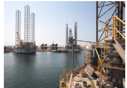
Before operations the rig ENSCO-104 went through a maintenance and upgrade procedure.
