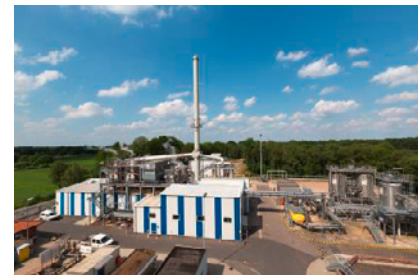
The steam flooding facility in Emlichheim produces hot steam that makes the crude oil easier to extract from the reservoir.
