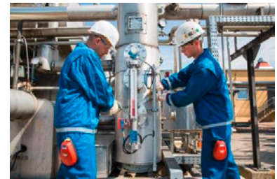
Working at the sour gas production plant at the site in Staffhorst.
